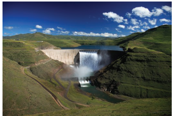
▼ Figure A.4.1. The Katse Dam in Lesotho
